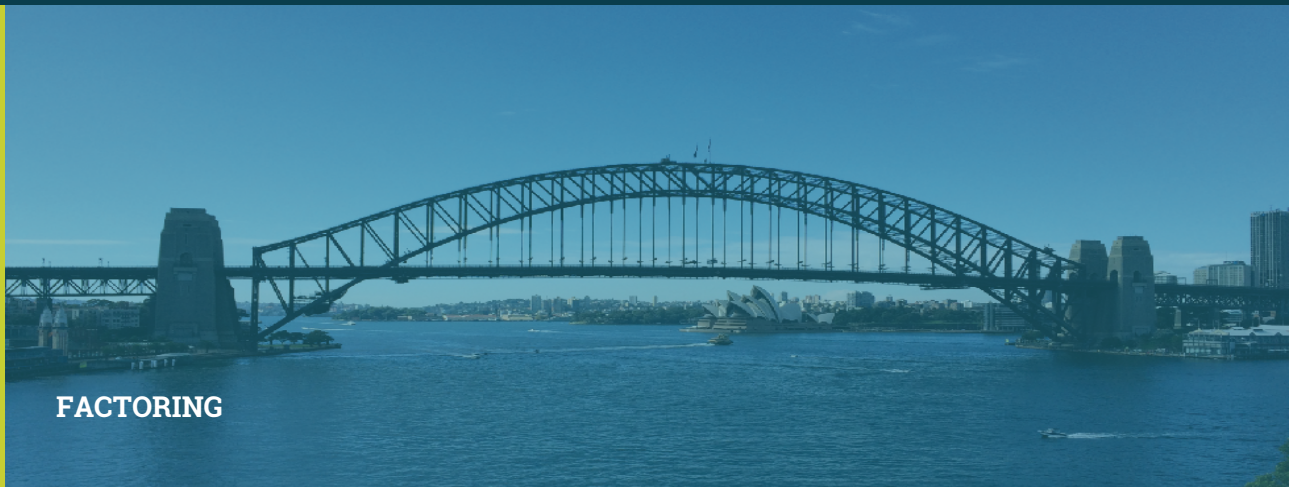
Figure 7.1 The Sydney Harbor Bridge is one of Australia's most photographed landmarks. It is the world's largest steel arch bridge with the top of the bridge standing 134 meters above the harbor. Can you see why it is known by the locals as the "Coathanger"?
