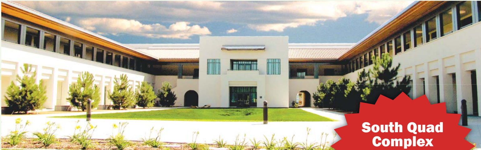
South Quad Complex will feature 32 high-tech classrooms and academic offices all powered by the new energy efficient Central Plant.
