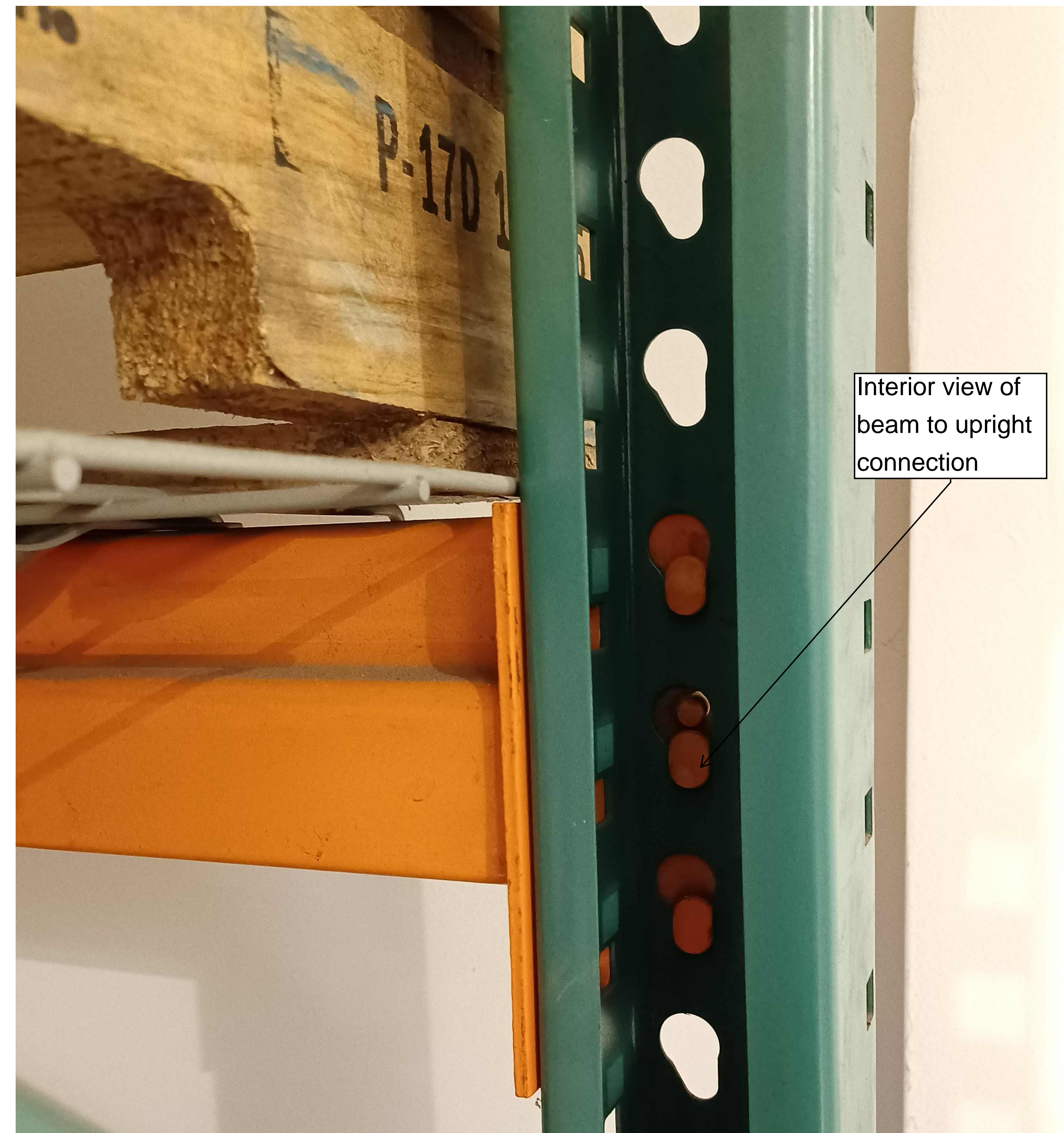
2 Interior view of beam connection to Upright
