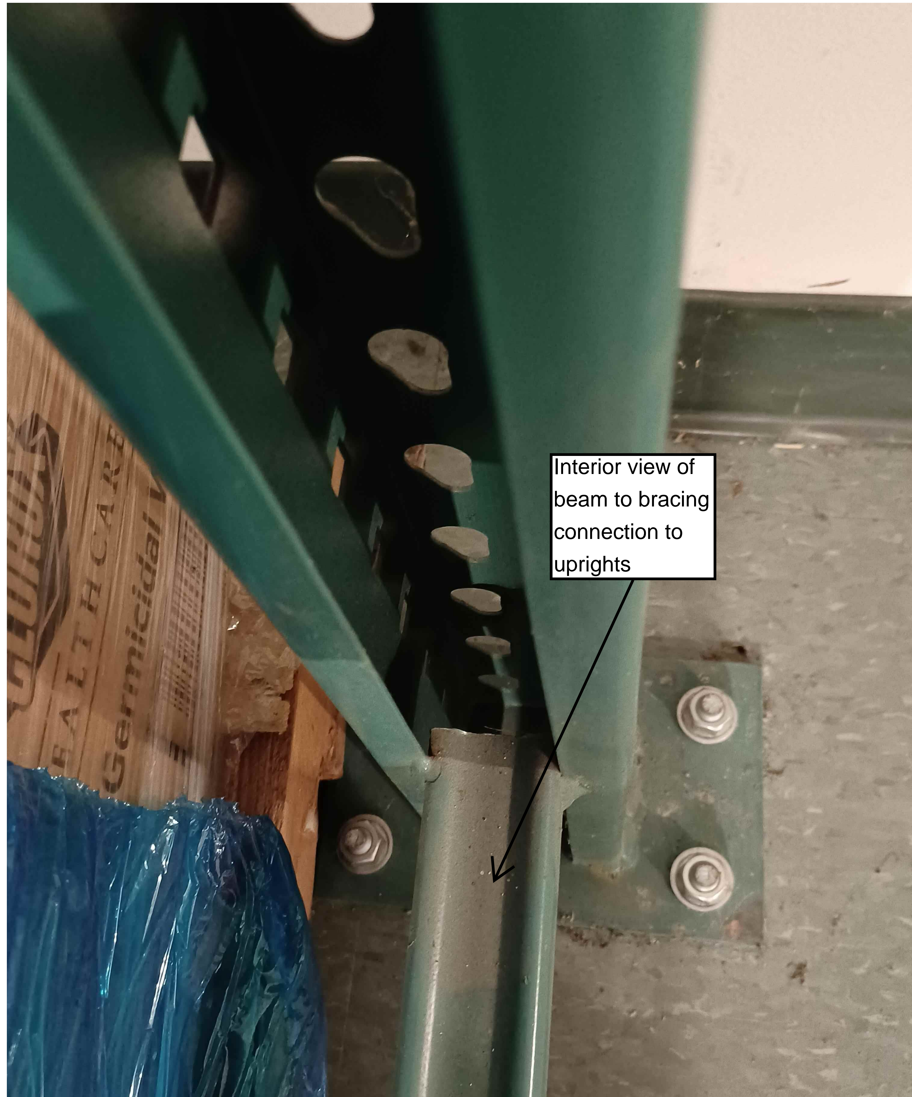
1 Bracing welded connection to upright
