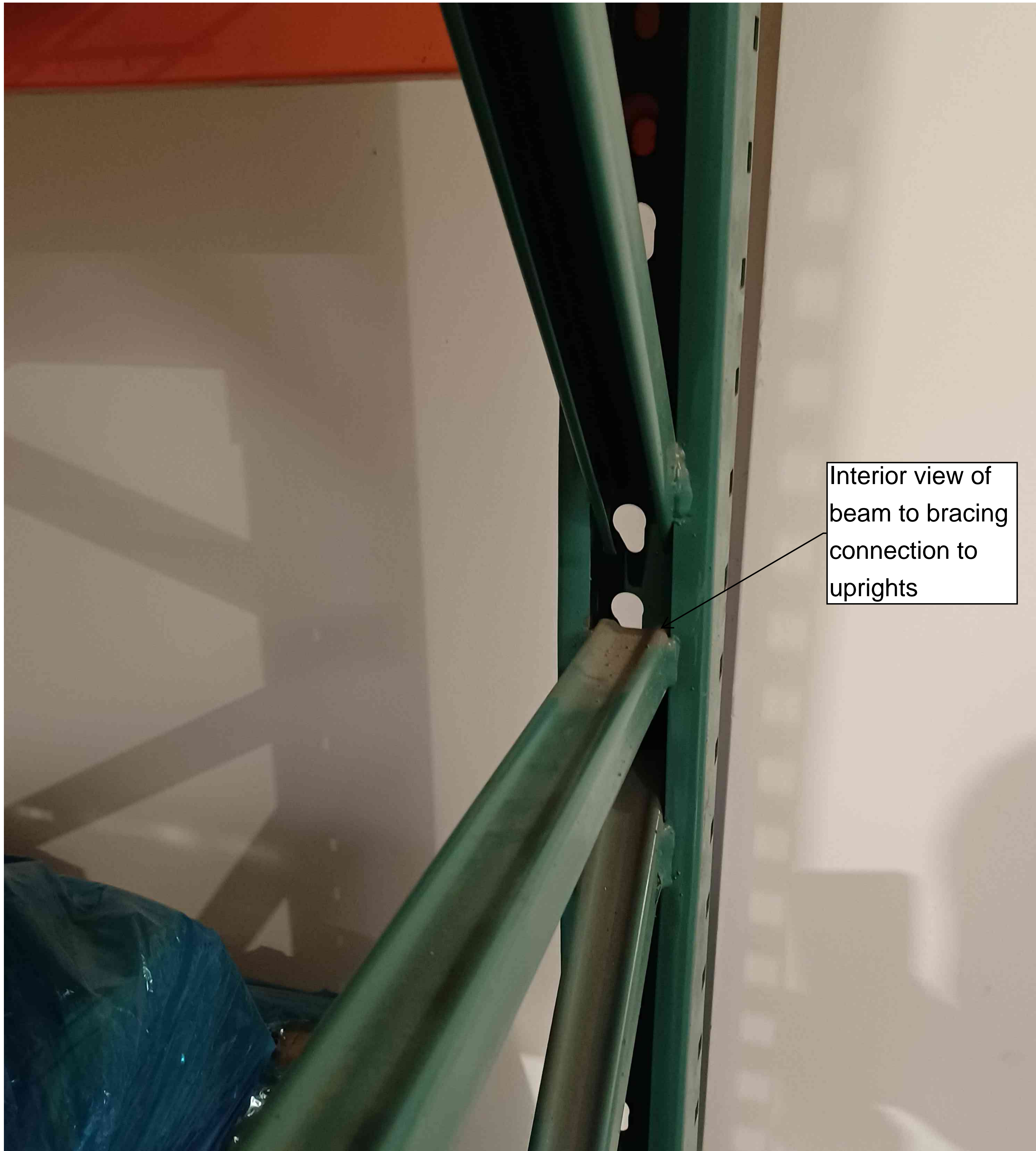
2 Bracing connection to uprights
