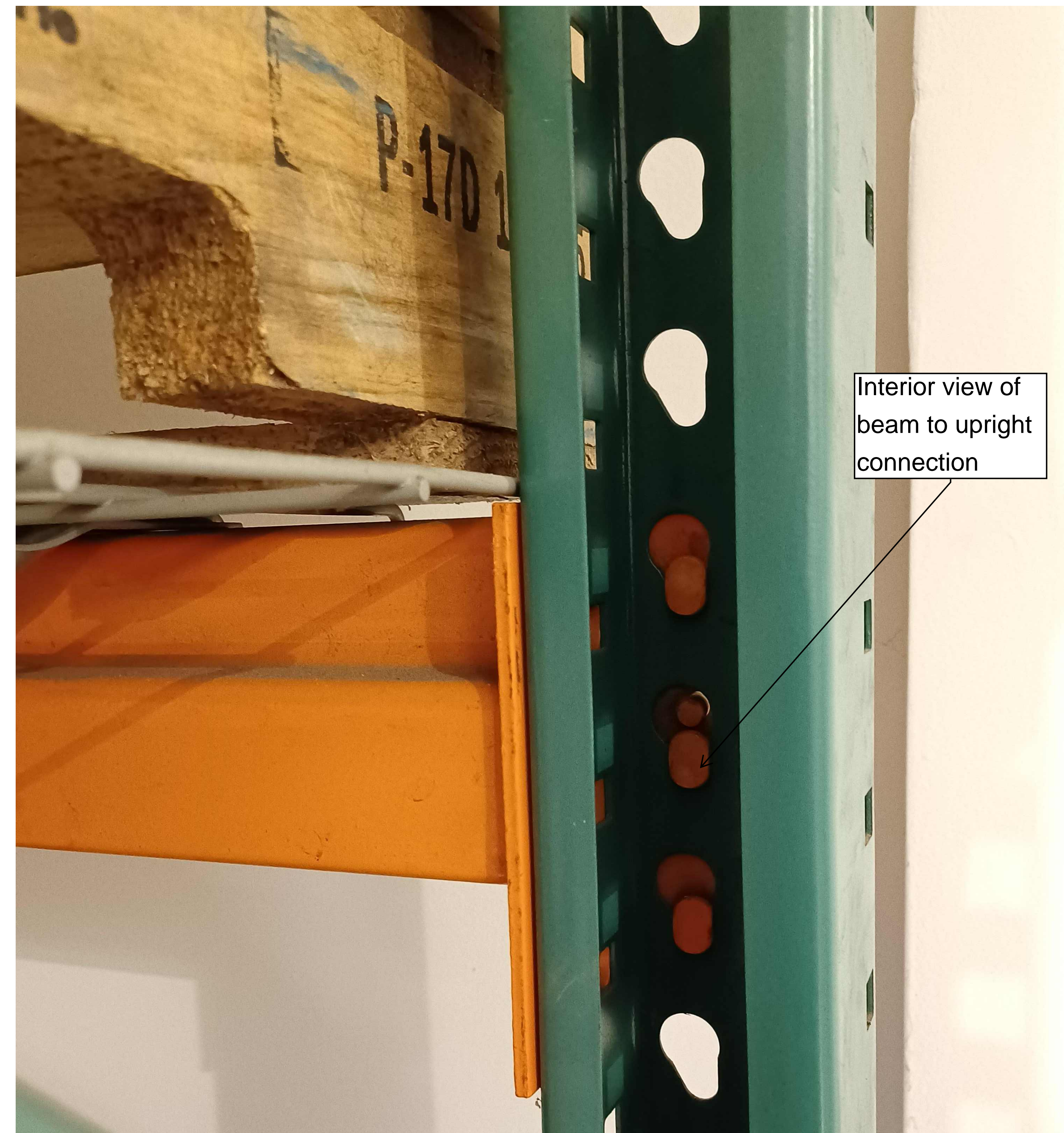
2 Interior view of beam connection to Upright
