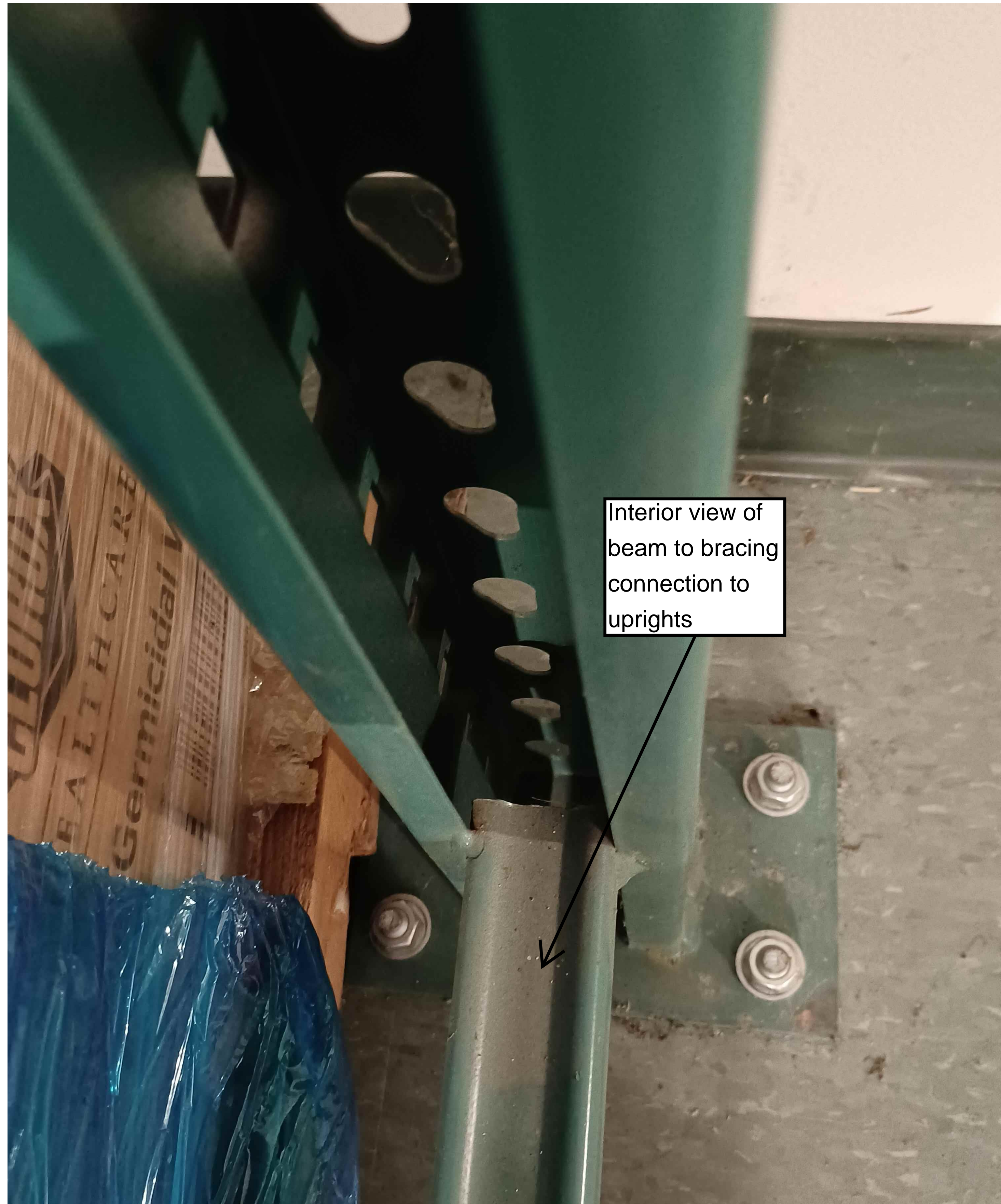
1 Bracing welded connection to upright
