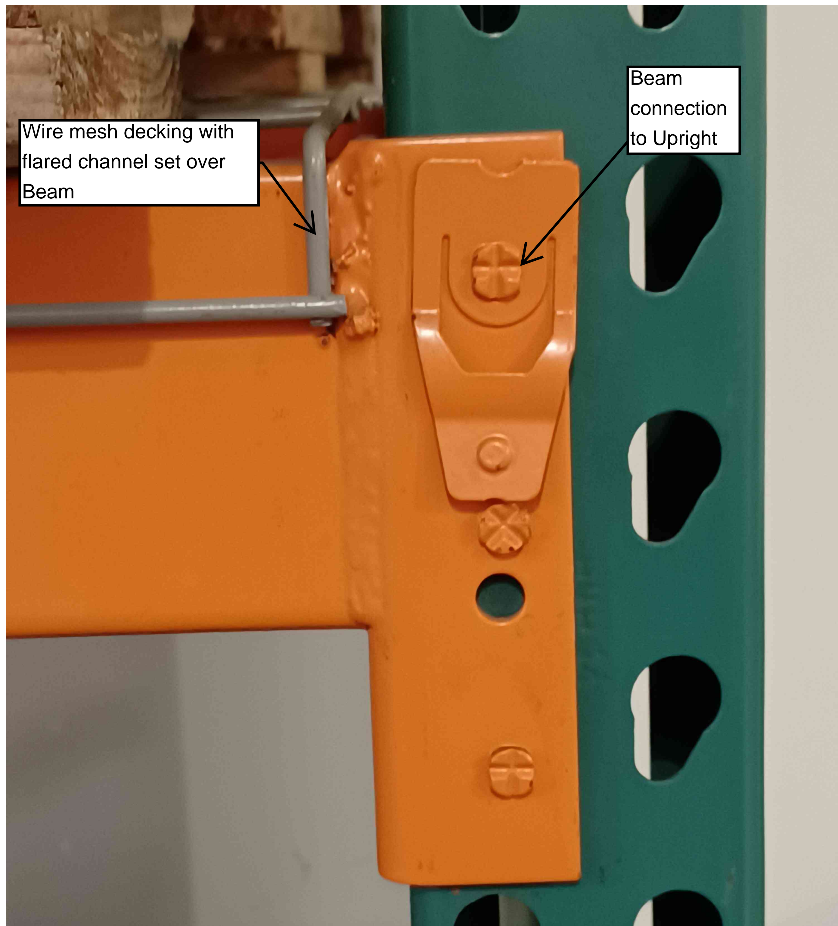
1 Beam Connection to Upright
