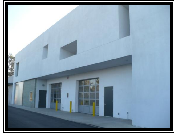
Central Plant – PCC
