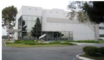
LAC Bldg. O Complex (back building)
