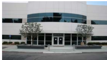
LAC Bldg. O Complex (front building)
