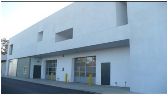
Central Plant – PCC
