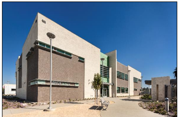
PCC Buildings QQ/RR—Electrical Program, Dyer Hall, and Lifetime Learning Center
