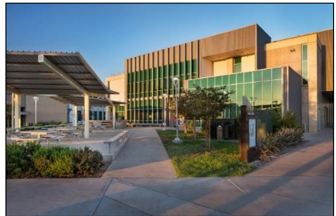
PCC Building GG—Student Services
